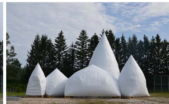
1 Day to Install a 100m 2 Instant House (2018)
